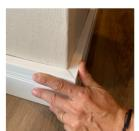
Cut the merging profiles in 45 degrees angle, when you are installing the corner pieces.
